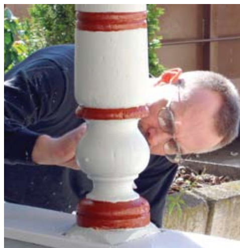
Providence St. Mary employee Clint Froke paints a pillar at Helpline, a non-profit emergency aid agency for the poor. Providence volunteers painted the exterior of the building in the fall of 2007.
